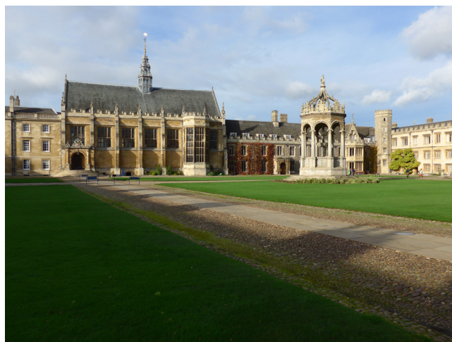
Figure 1 Great Court from K staircase
